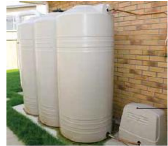
3 m 3 tank. Too small to have any meaningful impact and relatively high cost.
