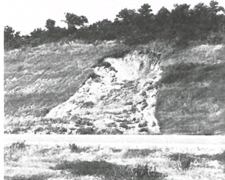
Figure 10-34 An earthflow in a roadcut near Dallas, Texas, shows the sharp scarp high on the slope and, farther down, the area of soil movement by flow. Compare with Figure 10-35. (Photo by C. W. Brown.)
