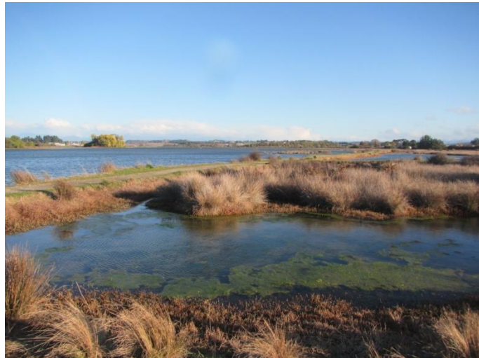
Photo 5. The causeway in the northwest corner of the Inlet, with a tidal pond in the foreground. Note dense algal growth; a larger culvert to enhance tidal flushing would be desirable.
