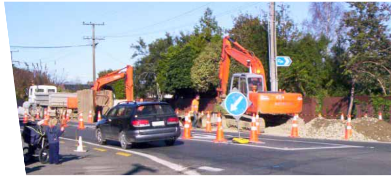
The stormwater upgrade being carried out on High Street, Motueka.
