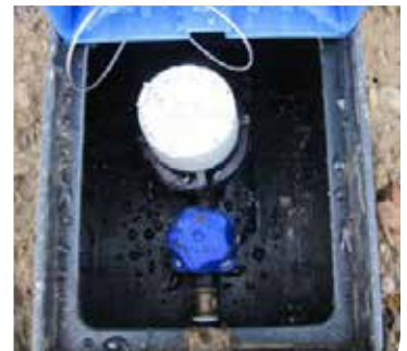
New water meter
