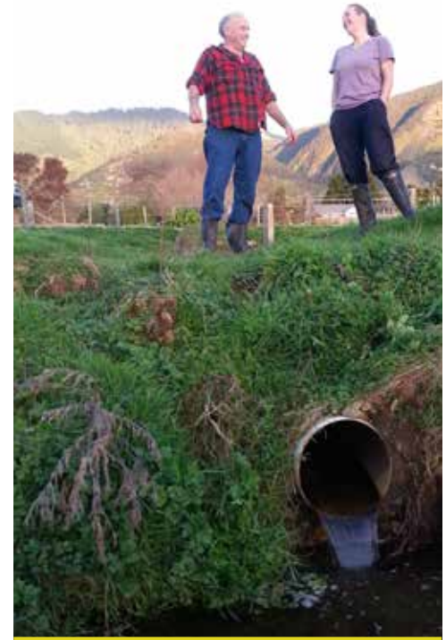
Ross and Helen Tullett, at Clifton showing us their culvert.
