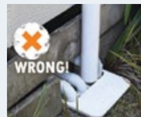
Downpipe going into gully trap
