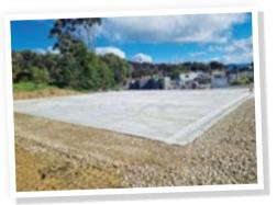
The new heavy-duty slab provides an improved base for the metal collection storage area and means products stored at Māriri will no longer be contaminated by dirt and mud off the ground before they're shipped out.
