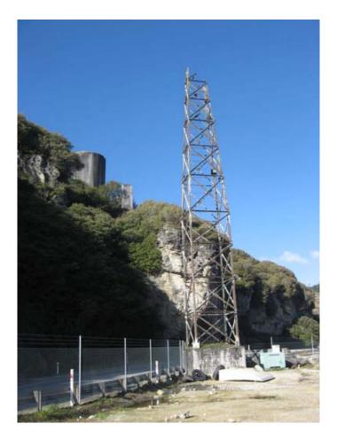
Photograph 19: Old conveyor support tower now used as a light tower
