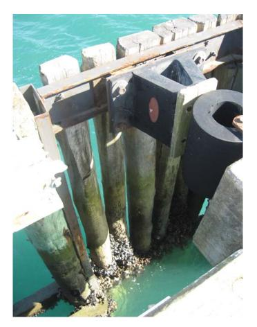
Photograph 5: Showing rubber components of fended system.
