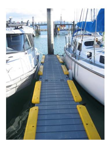
**Photograph 17:** Plastic floating marina – last section has partially sunk due to water leaking into it. Needs to be pumped out.
