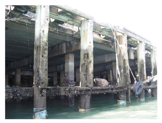
**Photograph 11:** Showing large section loss in horizontal timber member of fender system. Note: large rock sitting on timber – probably has fallen during loading of barge.
