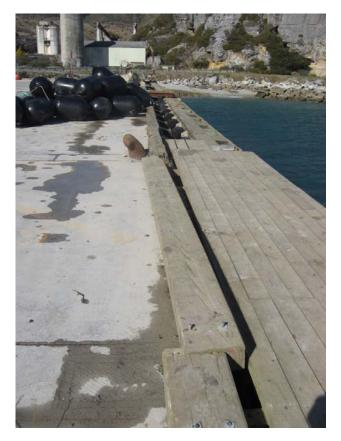
Photograph 3: Loose timber kerb at edge of wharf.
