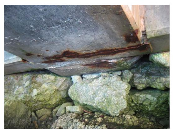
Photograph 9: Typical cracking and rust staining to underside of beam joint on landward side of wharf.
