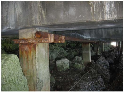
Photograph 10: Disused pipework and steel supports causing rust staining to concrete piles.
