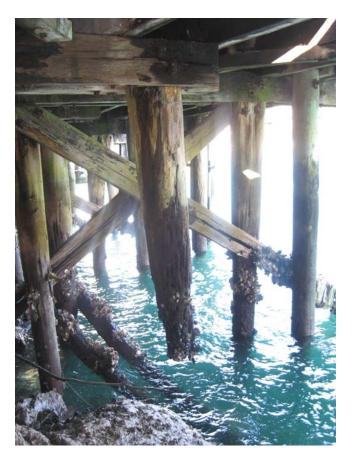
Photograph 15: Showing badly deteriorated pile that no longer reaches the water.
