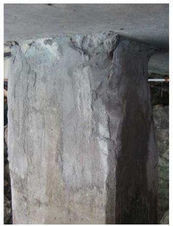
**Photograph 7:** Typical spalling of concrete at top of piles.
