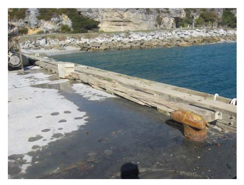
Photograph 4: Damaged timber kerbs.
