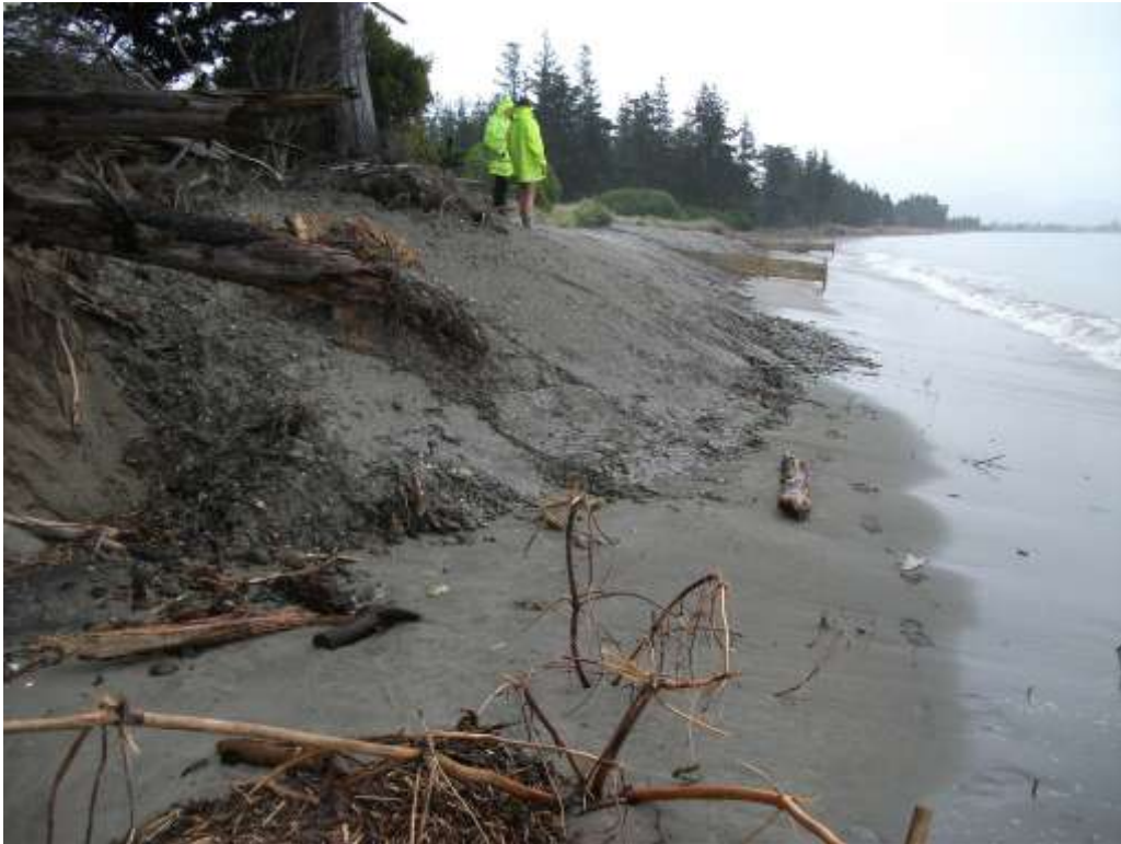
Photograph 1 Completed emergency works as at 6 July 2011
