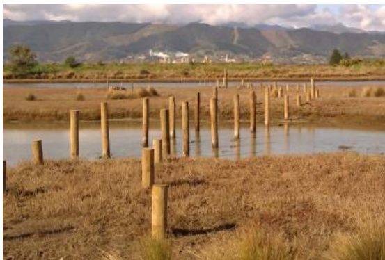
Board walk piles, Nieman Creek
