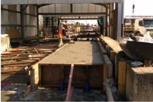
End deadmain 14 tonne concrete block
