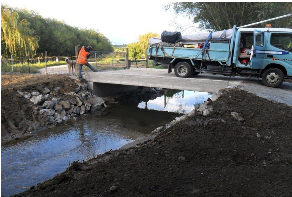
Figure 8.1 - New bridge on Ellis Creek
