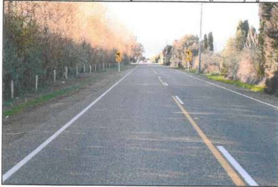
View facing eastwards approaching intersection, showing advisory sign.
