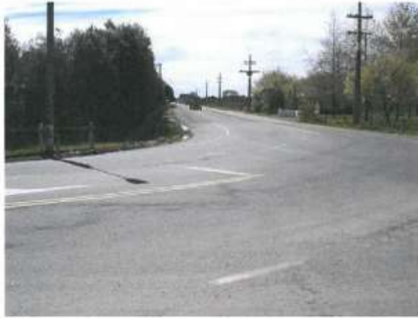
Photo 5: Ponding adjoining Existing Intersection
