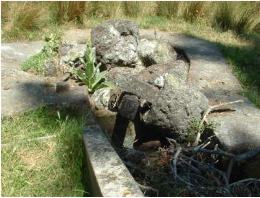
A key hole shaped plunge dip, filled with rubble.
