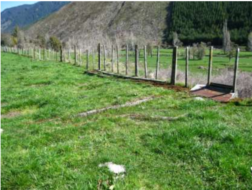
The sheep went into the dip from the metal slope. The concrete rim is visible and the drainage pad is present under the grass.
