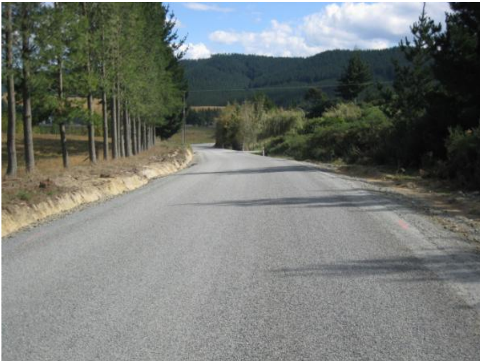
Sealed section awaiting road marking and trimming of the shoulder batter
