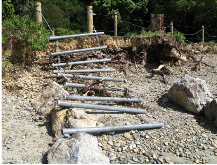
December 2008 beach accessways washed away
