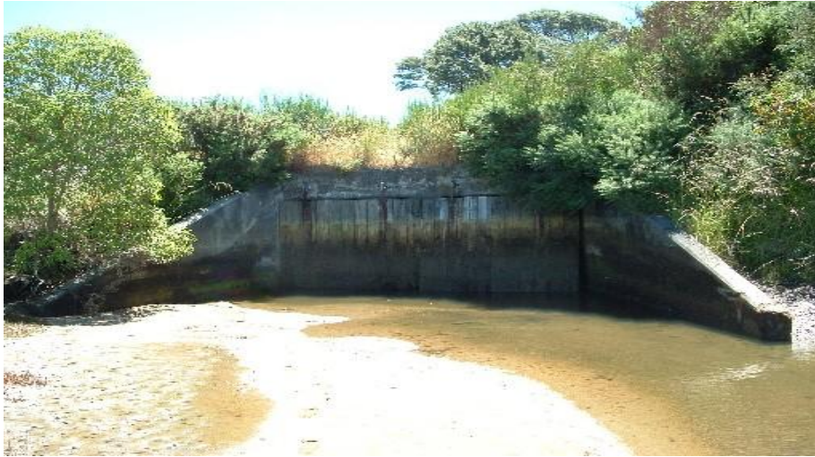
Figure 17: Wai Atua Stream Tidal Flap gate.
