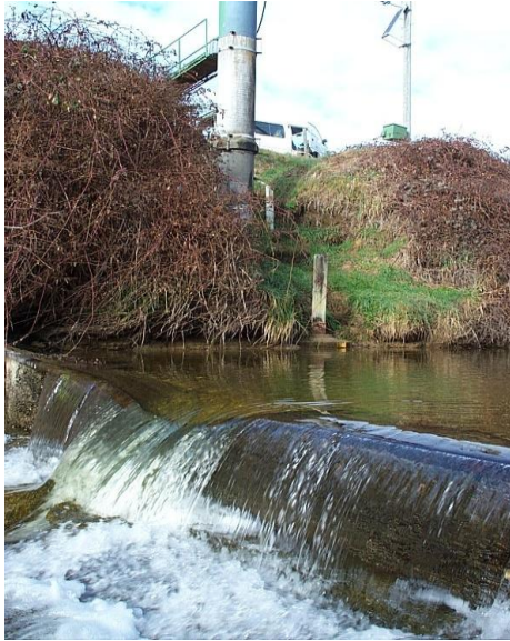
Figure 19: Tadmor River, TDC Hydrology weir
