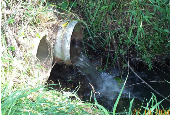
Figure 5: Reservior Creek Culvert, tributary Kareti Drive (now removed).
