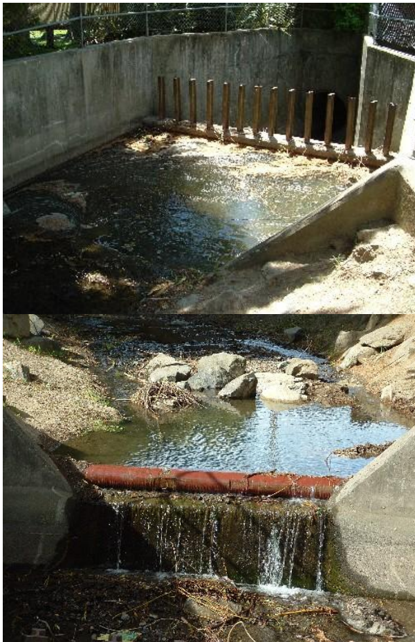
Figure 2: Reservoir Creek, Marlborough Terrace Easby Park.
