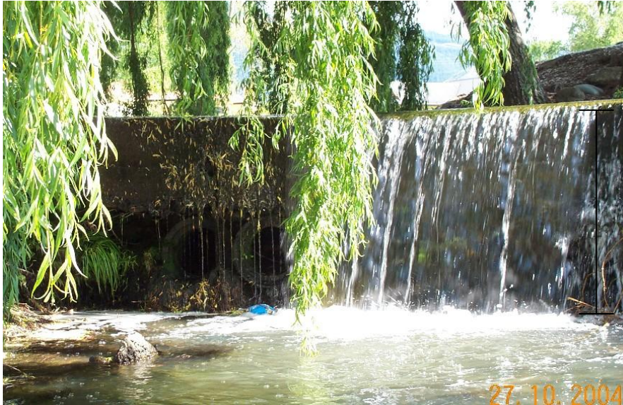
Figure 11: Reservoir Creek Concrete Ford downstream Templemore Pond (Scale 1.0 m).
