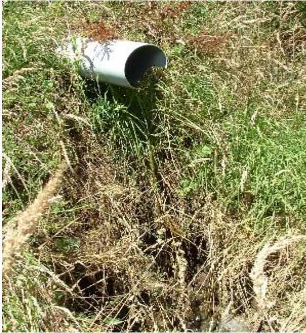
Figure 7: Reservoir Creek, Walkway
