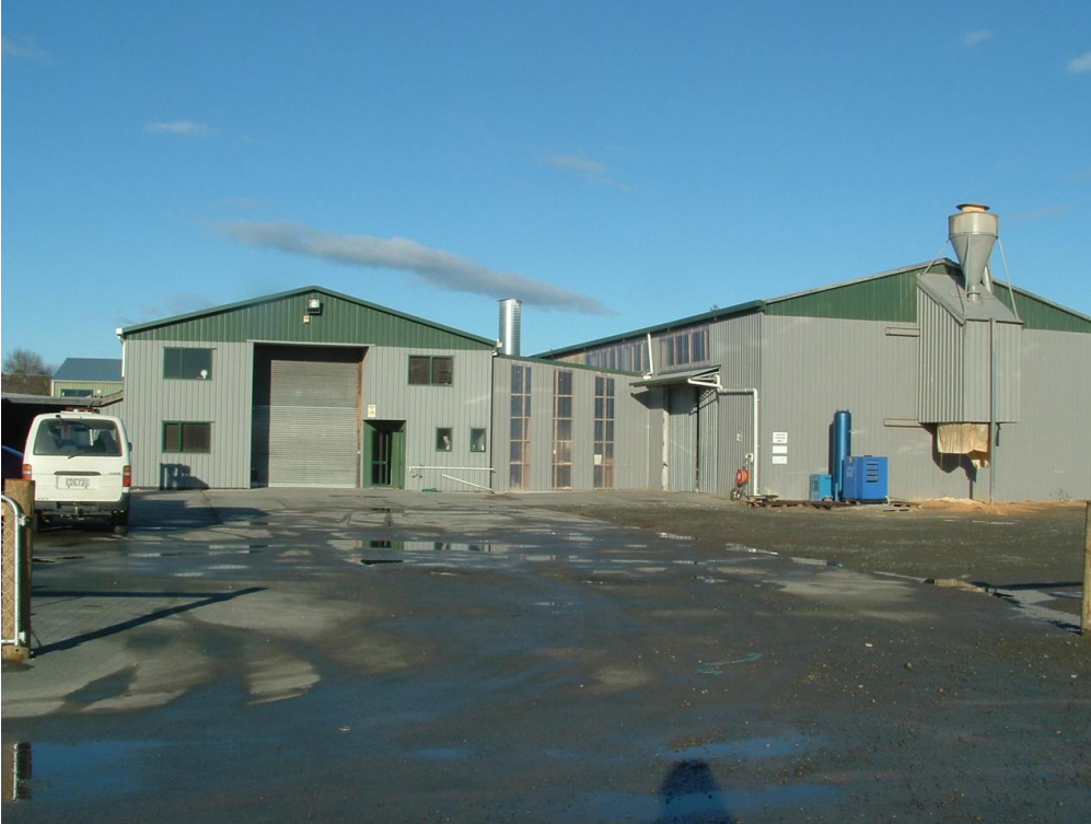
a) Photo showing the subject building, formally used as a packhouse
