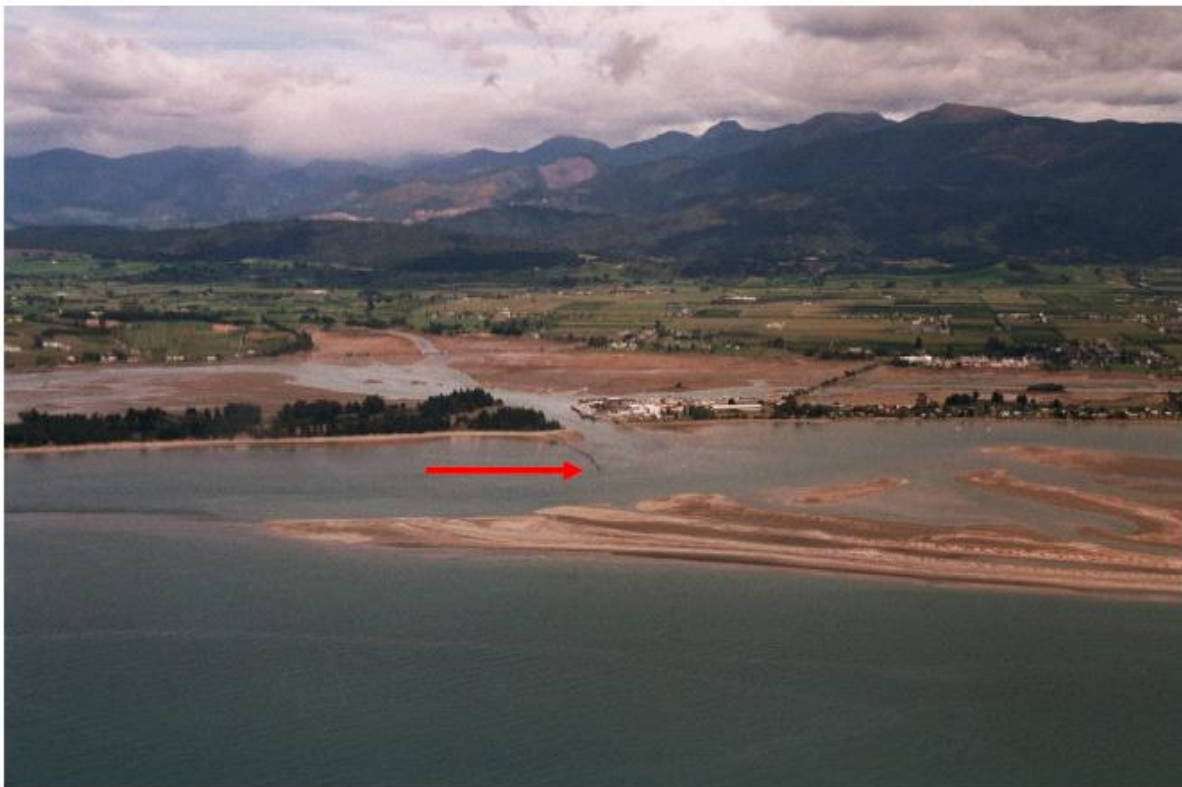
Photograph 1: Location of wall as viewed from Tasman Bay (photo sourced from application)
