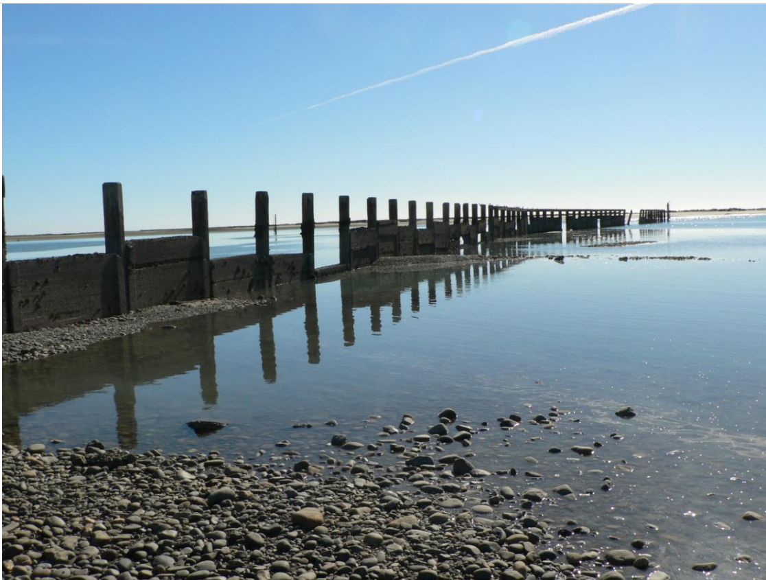
Photograph 2: Existing state of repair of training wall viewed from Jackett Island
