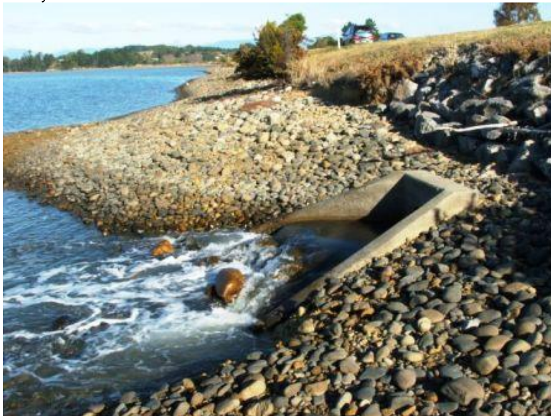
Figure 5: Weka Road Culvert
