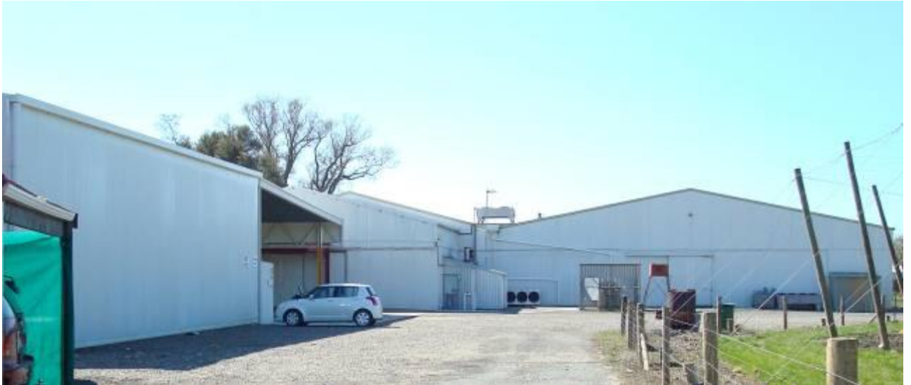
Photograph 7: Main car parking area at south end of coolstore
