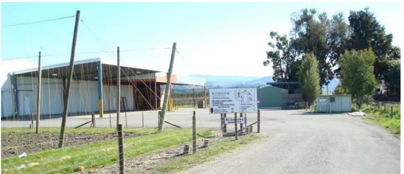
Photo Eight: Overflow car park from pump shed back to ward green shed. Traffic signs. Packhouse and original coolstore at centre left.
