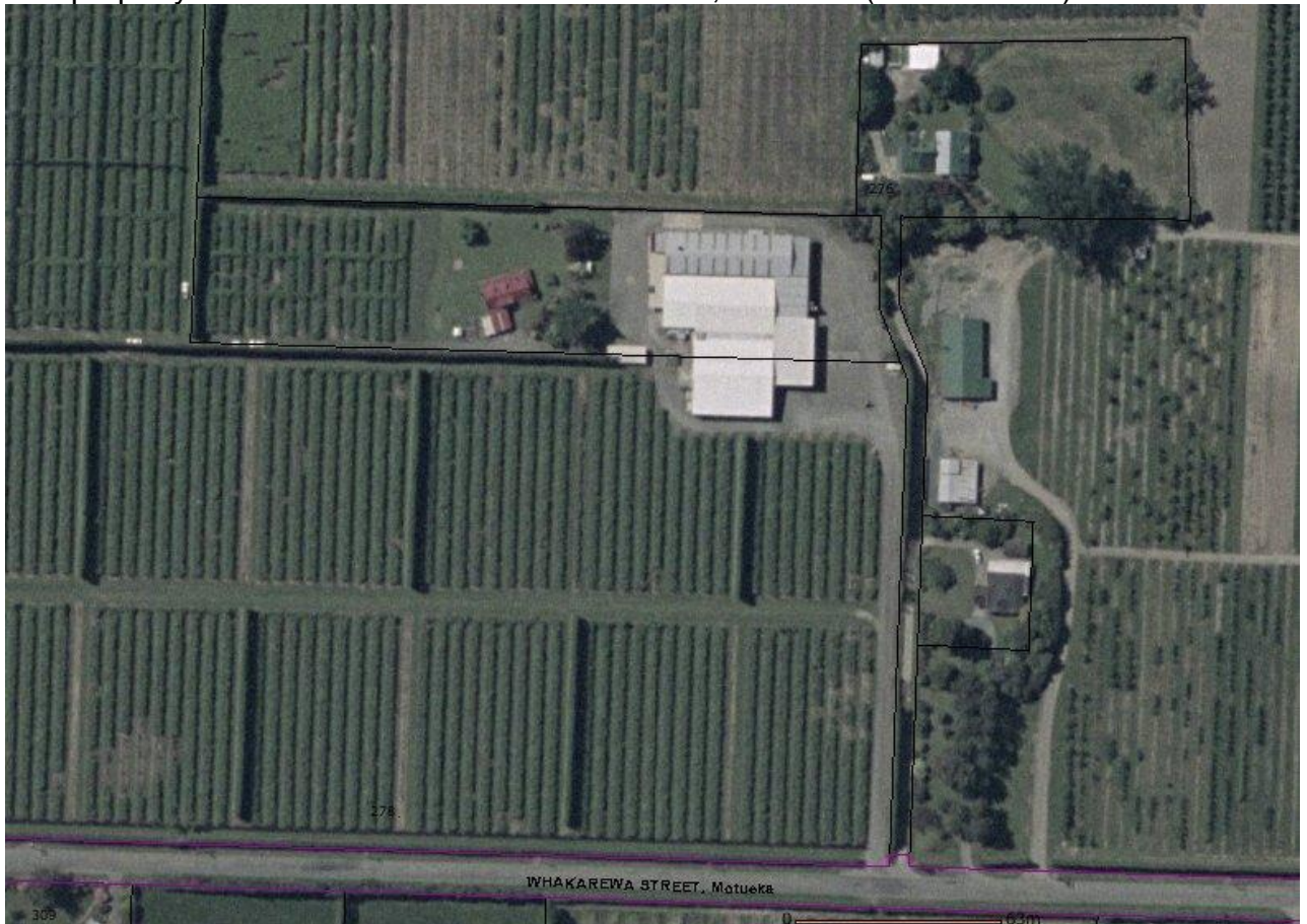
Photograph 1: Explore Tasman aerial photograph of Ngatahi coolstores prior to building consent BC 071627 NEW COOLSTORE AND CANOPY (COMPONENT E)
