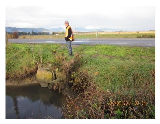
Photo 2: Location of where a platform or culvert extension and reclamation may be required to achieve adequate width.
