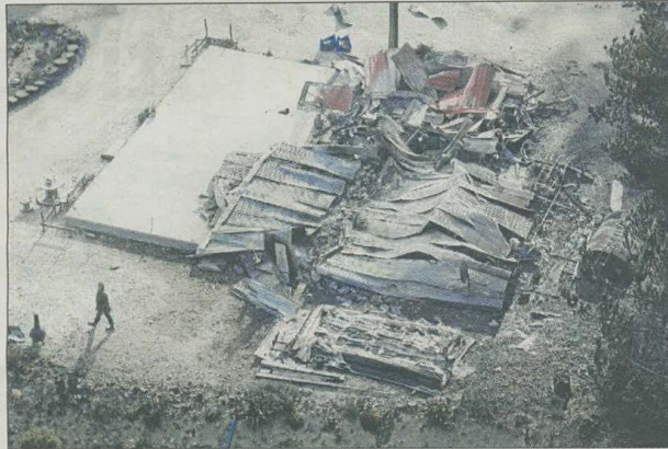
Access issues: Dangerous access mean this Glenhope home could not be saved by fire fighters in 2009. Photo: MARTIN DE RUYTER.
