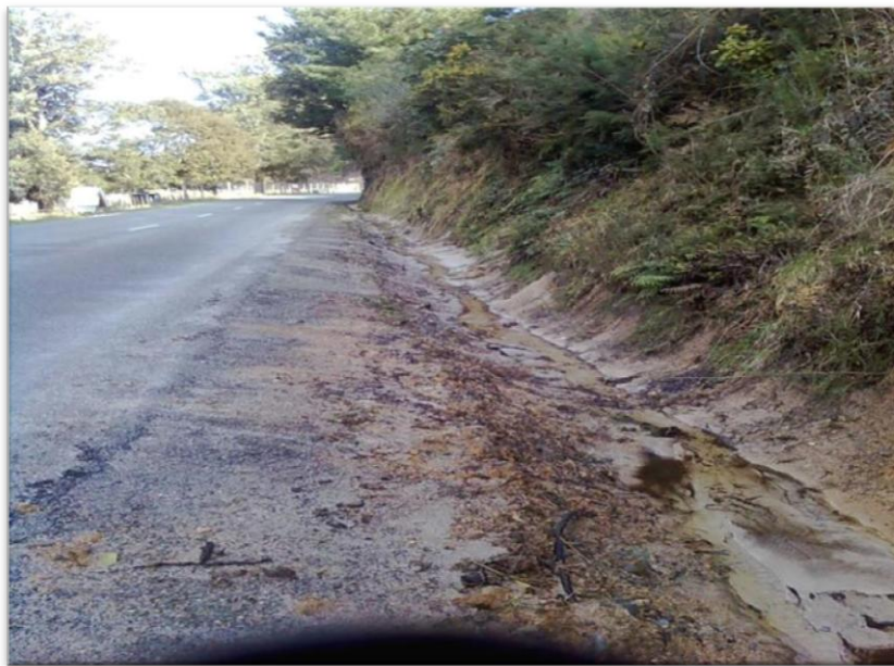
Motueka River West Bank Road Drain Cleaning
