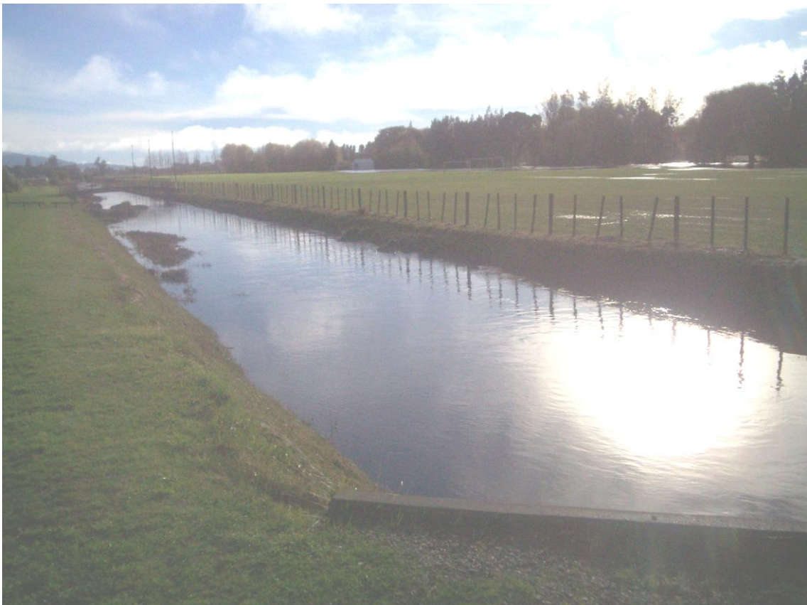
Woodland Drain after gates commenced manual opening
