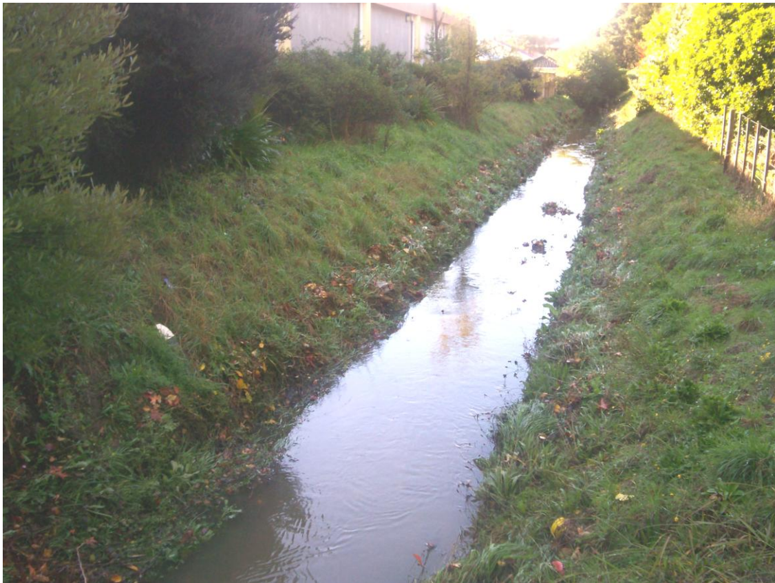
Backup of Floodwaters outside New World (Head of Woodland Drain)
