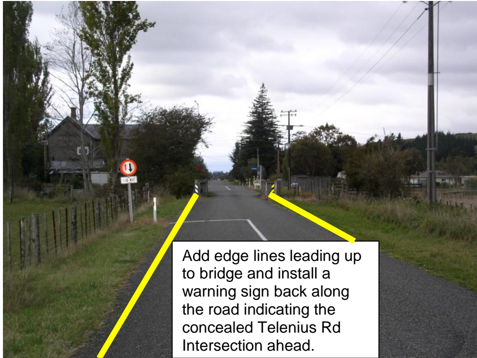
Telenius Bridge on Higgins Road – Looking North
