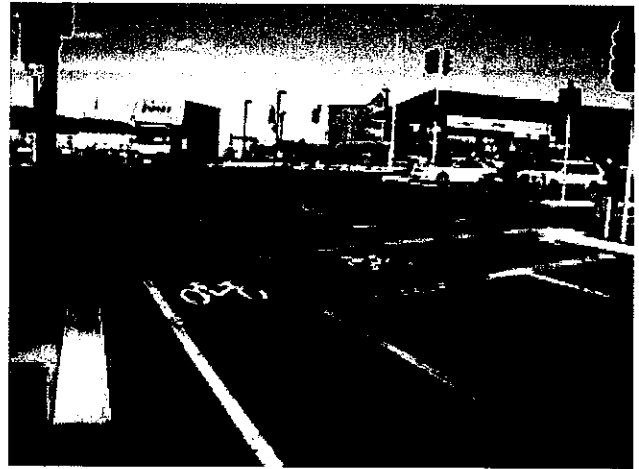
Advanced stop box for cyclists at an intersection in Christchurch
