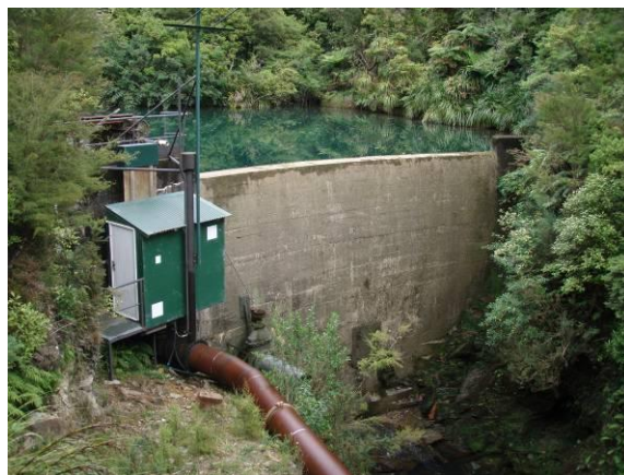
Above: Electric Waters Dam on the Onekaka River (January 2009)
