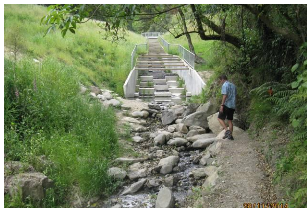
Reservoir Creek at the Reservoir Spillway (Nov 2014)
