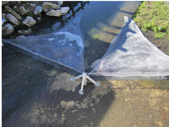
Jimmy-Lee Ck downstream of Wakatu Dr and piped section. Left: View upstream from near 35 Beach Rd and Right: close-up of coarse rubbish traps (both photos from May 2011)
