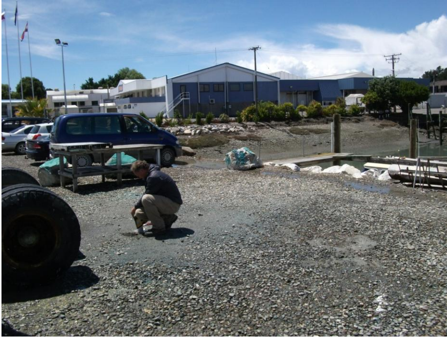
Photo 12: Motueka Slipway showing Paint Fragments in the Gravels and Paint Spray on Adjoining Rocks
