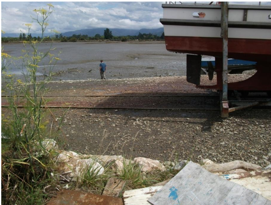
Photo 13: Waitapu Bay Slipway with Paint from Vessel Water Blasting Shown Near the Beach Cradle and on the Ramp and Beach
