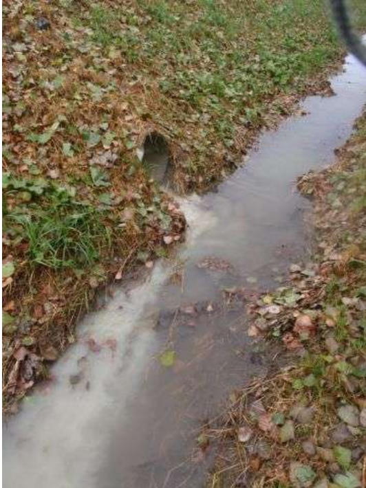
Figure 5a Discharge to Borck Creek downstream Gladstone Road on the Railway Reserve
