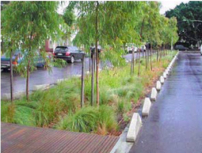
Figure C3a Rain garden in a residential street
