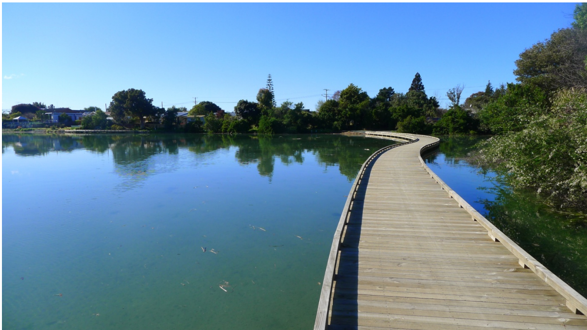
Inlet Walkway, Motueka
