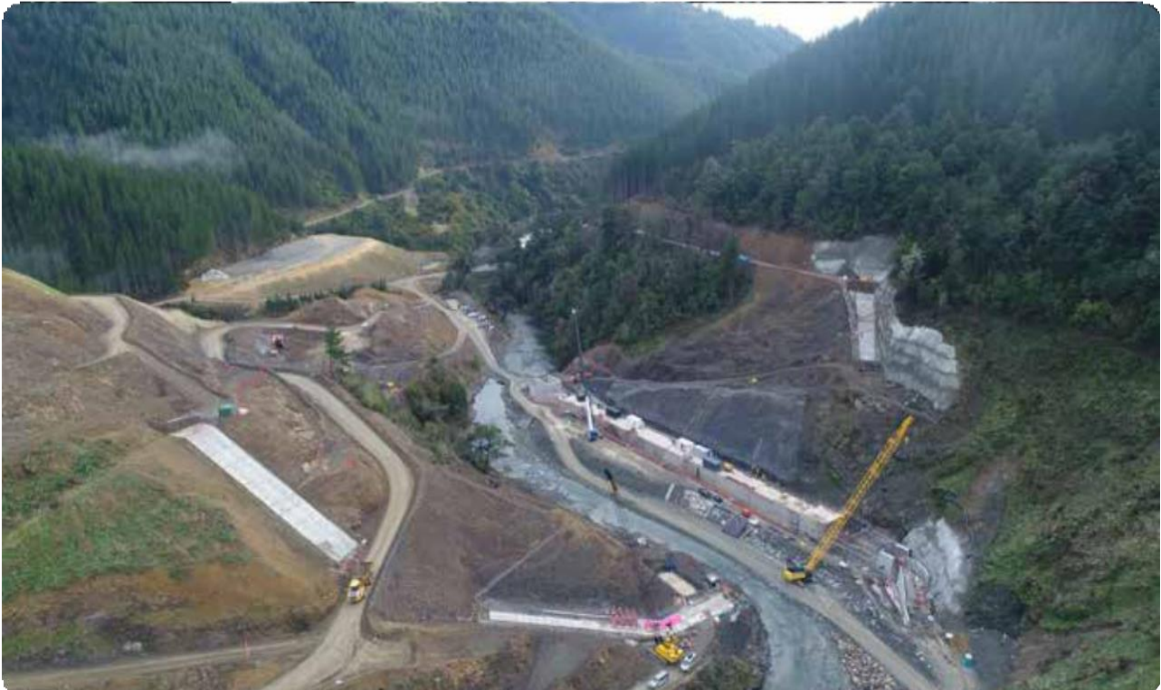
Next Step: Divert river to enable main dam construction
