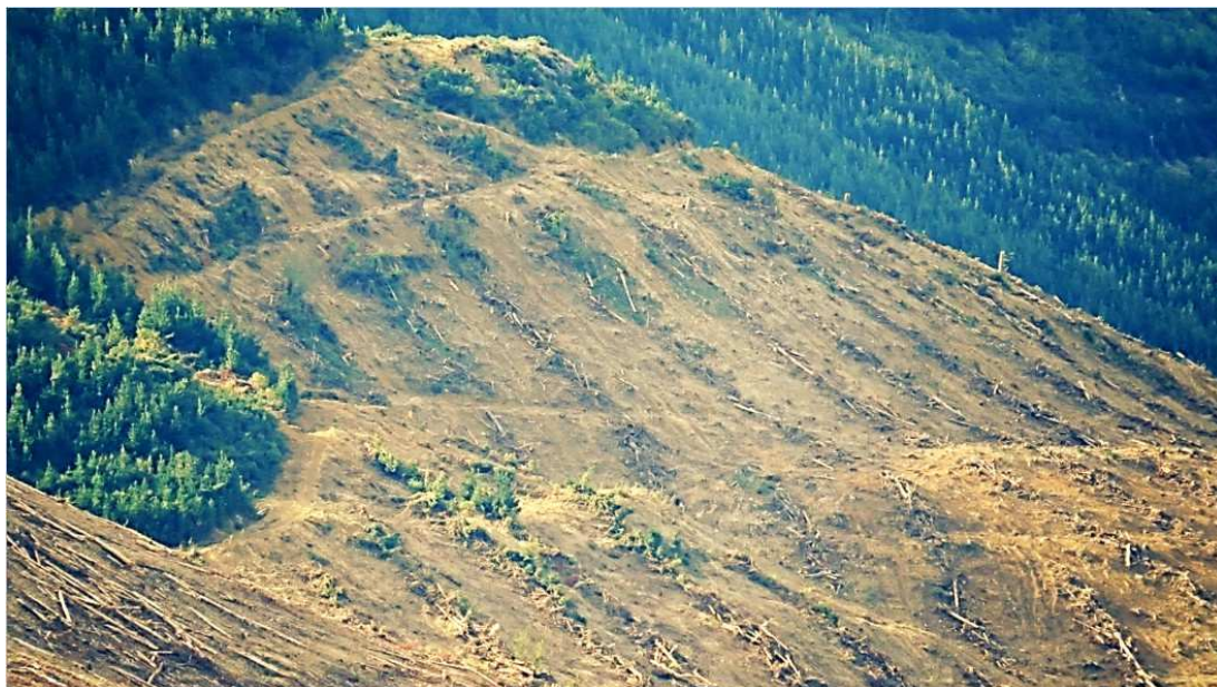
Figure 4-2: Wind-rowing pine slash down the slope can exacerbate soil erosion. This practice enhances the runoff velocity and thus erosive energy down the slope during rain events. Wind-rowing across the slope causes the water to slow as it passes through each wind-row reducing velocity and erosive energy. [Photo by M. Gibbs]The effect of land use/management is captured by the CSSI technique, and the results
