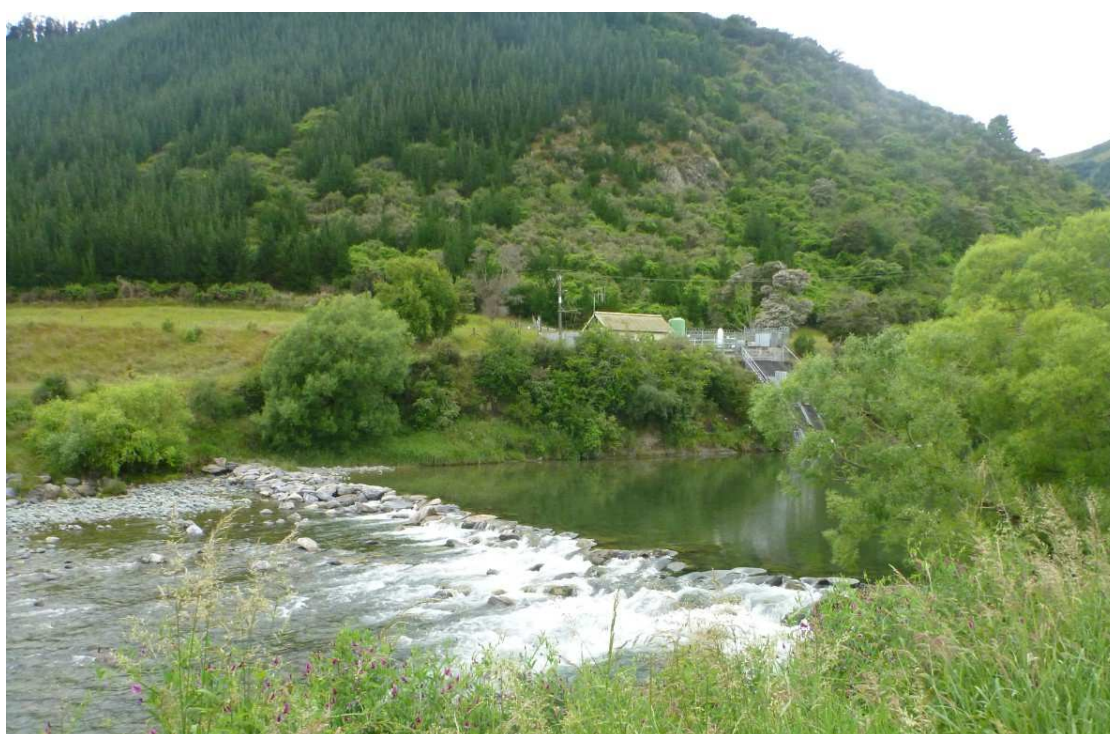
Figure 4-4: Waimea East Irrigation weir on the Wairoa River downstream of the Lee River (Site 9). The pool behind the weir acts as a sediment trap enabling fine sediment from further upstream to settle along the banks. There is also an area of native forest regrowth on the steep, northern banks, which may be a local source of the high proportion of native forest sediment class found at this site.
