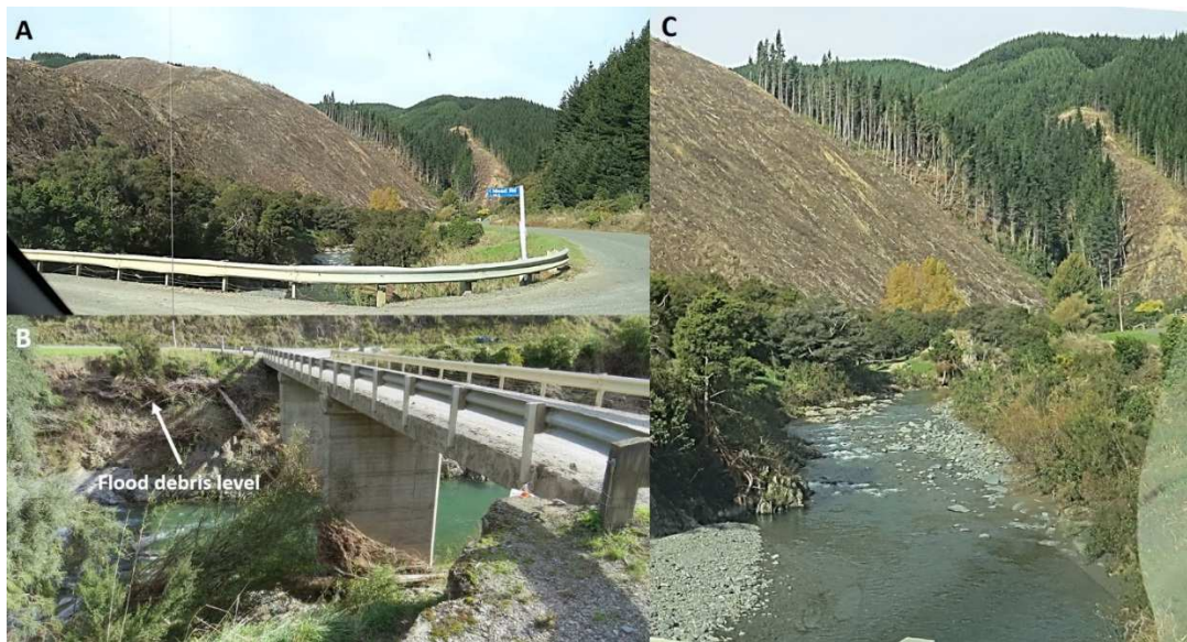
Figure 4-1: Lee River sampling Site 4 at Mead Road-Lucy Road junction at the bridge. A) View of the extent forest harvest upstream of this site; B) level of flood debris beneath the bridge; C) view upstream from the bridge showing the cobbled and rocky nature of the Lee River bed. Sediment samples were collected from the deposition zone on the true right bank. [Photos by M. Gibbs].
